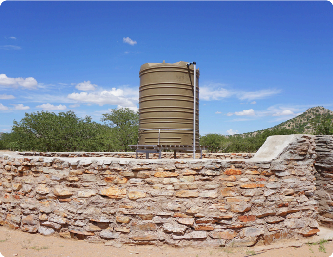
A water tank surrounded by an elephant-proof wall in Hobatere Concession, Namibia.
